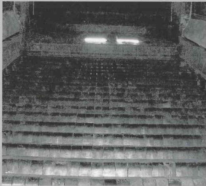
Grate bars in waste incineration
